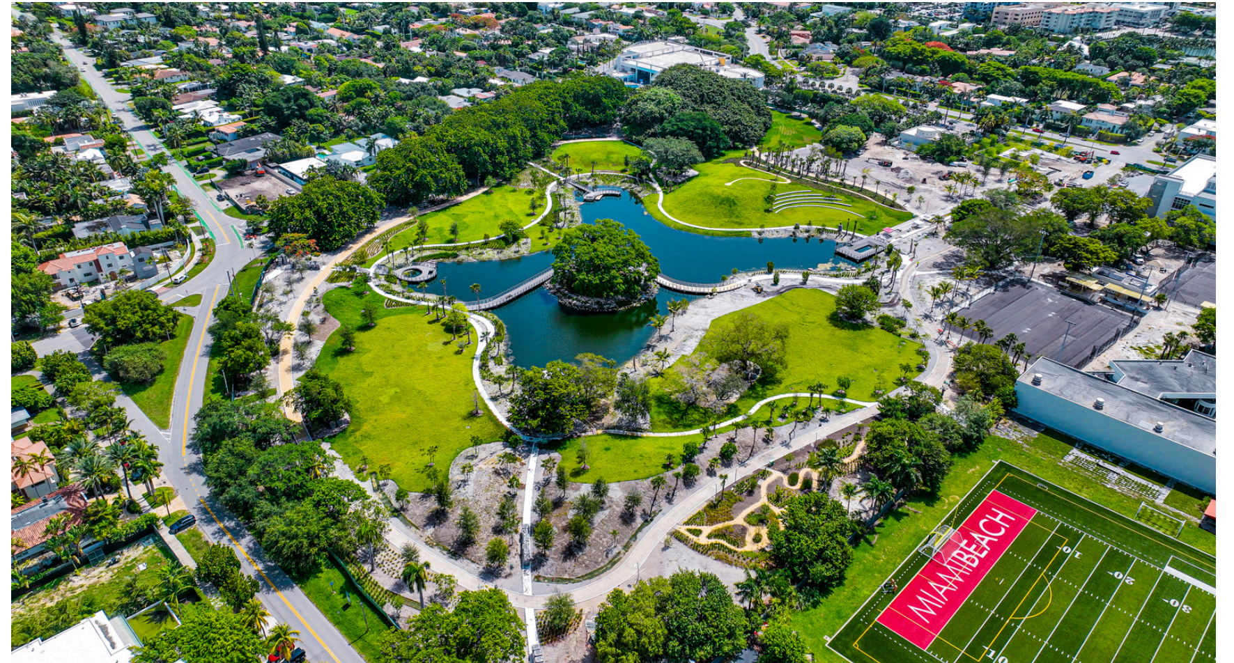
Aerial view of park near completion
