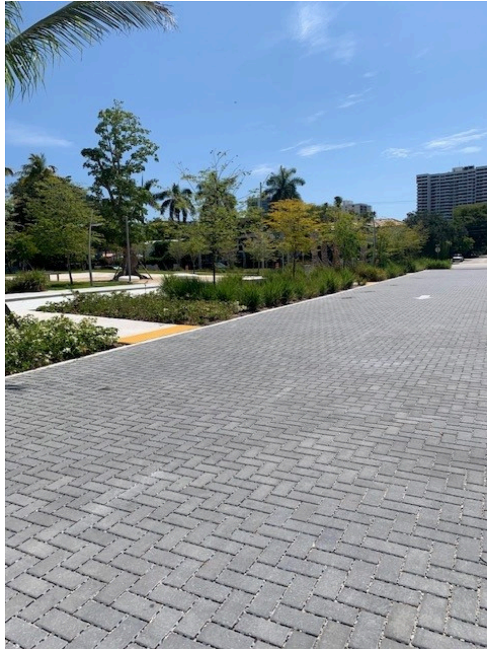
Permeable paver system in the parking lot
