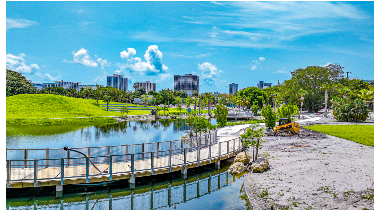
Portion of the park during construction near project completion
