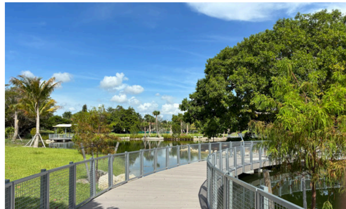
Walking path bridge on the retention lake
