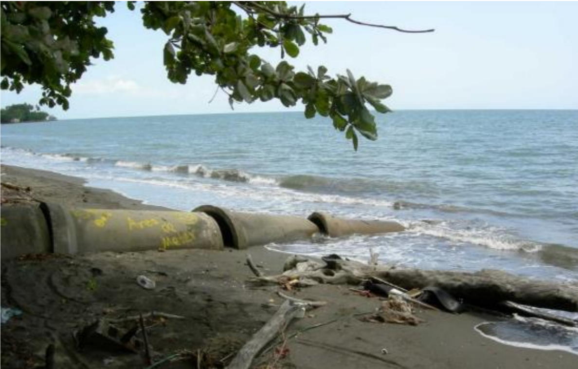
Existing stormwater outflow pipe on site
