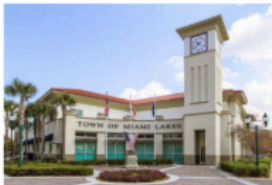
Miami Lakes Town Hall 25,000 sq ft 2013 Municipal building
