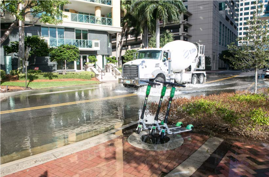
Sunny-day flooding in Fort Lauderdale disrupts travel and services and causes damage to infrastructure.
