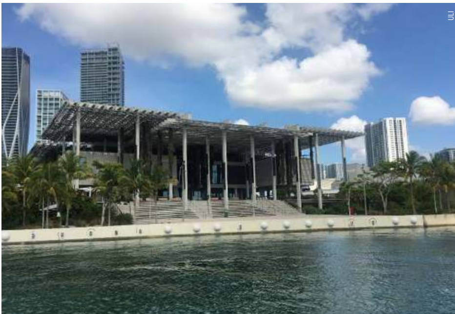
The Pérez Art Museum's first level is elevated more than 20 feet to protect art from flood risks.
