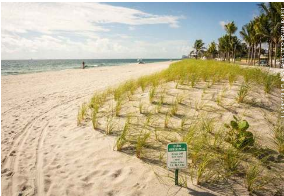
Extensive dune rebuilding efforts were conducted in the aftermath of Hurricane Irma in 2017. The Broward County Shore Protection Project placed 413,000 cubic yards of sand along the 8.9 miles of shoreline reaching north from Fort Lauderdale, according to the U.S. Army Corps of Engineers.
