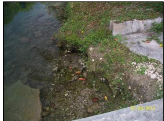
Canal Erosion on SW 194th Street
