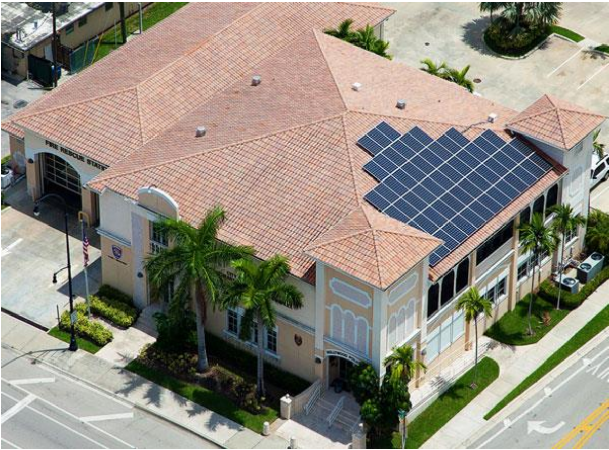
Fire Station 74 Solar Array
