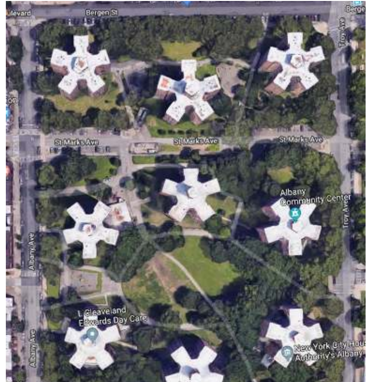
NYCHA – Albany Houses after roof coating in 2018
