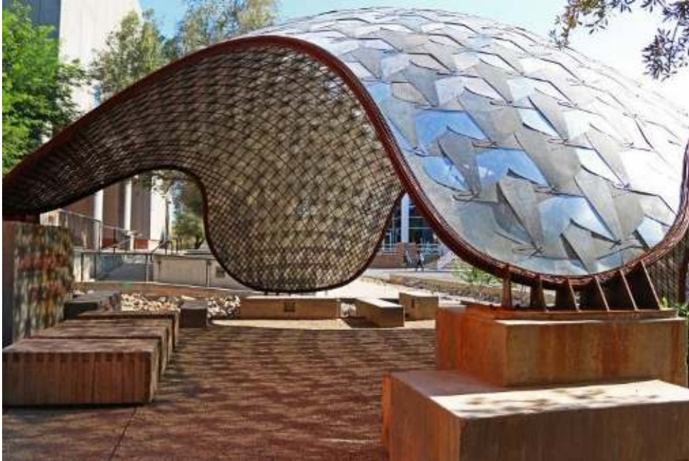
Shade structure at The University of Arizona's College of Architecture, Planning, and Landscape Architecture (AZ Daily Wildcat, Ian Green)
