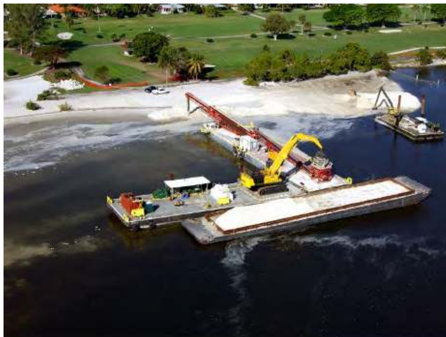
Fill being placed and graded at Snook Islands, 2004 ©J.E. McAmis Inc.
