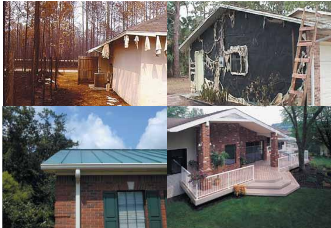
The top left photograph shows the melted soffits and soffit vents on a house that has survived a wildfire. These melted soffits could have allowed embers to enter the eaves of the house. The bottom left photograph shows a house with noncombustible metal soffits, roofing, and gutters, and masonry siding. The top right photograph shows a house with vinyl siding that has melted in the radiant heat of a wildfire. The bottom right photograph shows a house with fire-resistant plank and masonry siding and melt-away vinyl railing that will fall away and not cause a fire hazard to the house. Photos: FDOF (top row), USFS (bottom row)
