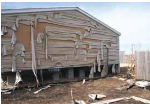
Even from 100 feet away, radiant heat from a wildfire can melt siding and contribute to ignition of the exposed wood sheathing. Photo: Texas Forest Service
