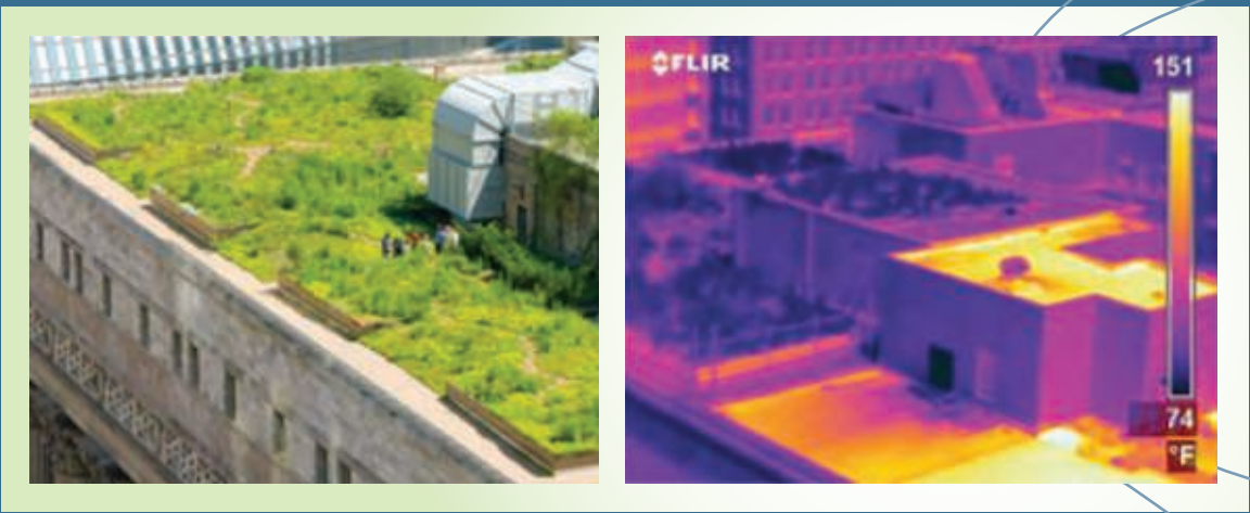
This visual shows the green roof on Chicago’s City Hall juxtaposed with the traditional roof of the county building next door, where temperatures are approximately 75°F warmer.
