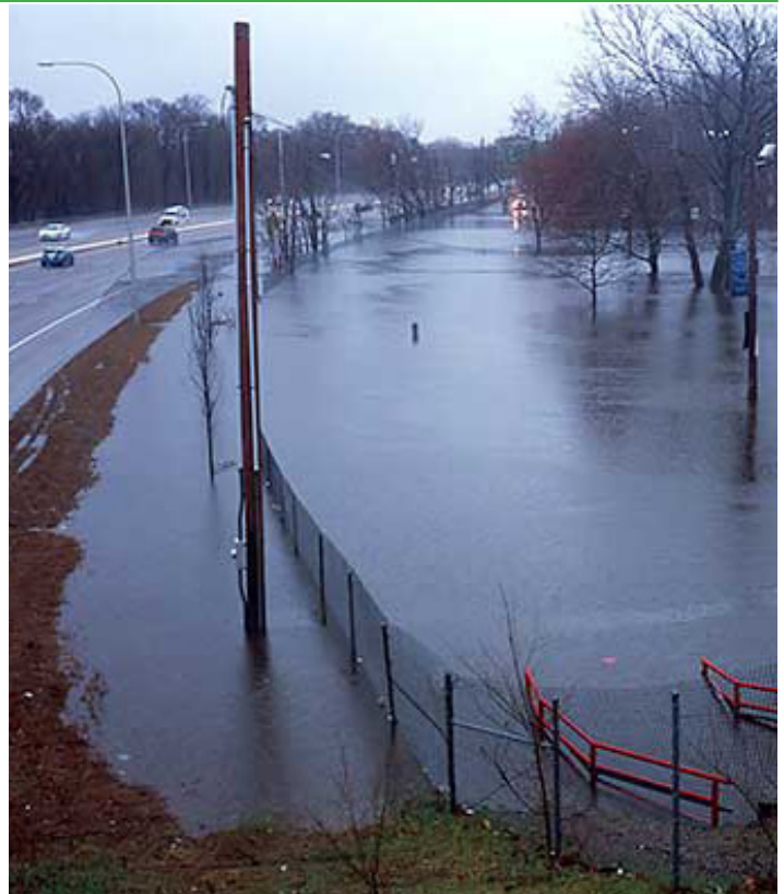
Merino Park from the end of the Footbridge. The river continued to rise after this photograph was taken on March 30, 2010 and later that day the eastbound side of Route 6 east was closed due to the water that was already starting to block the highway. Photograph by: Bruce G. Hooke.
