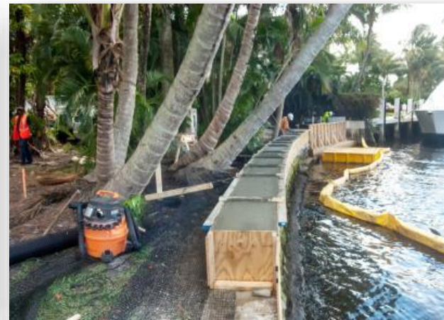
Raised Sea Walls
