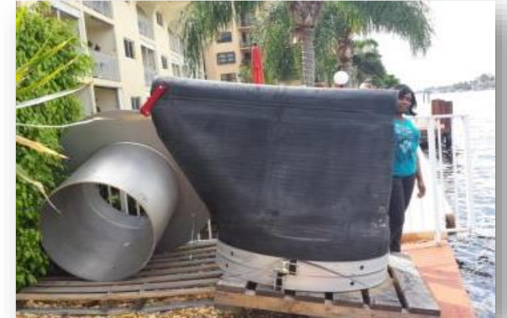
Storm system Improvements
