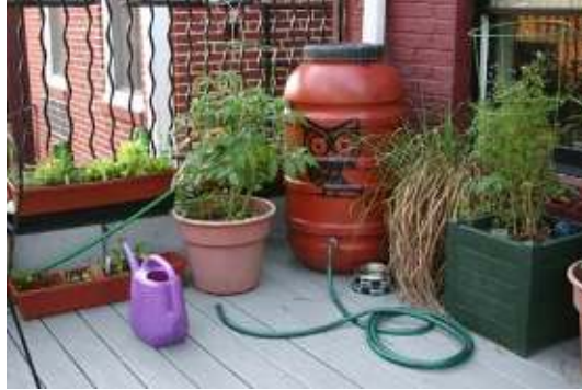
Household-scale green infrastructure can include rain barrels, which collect rainwater to temporarily reduce flow to storm drains.
