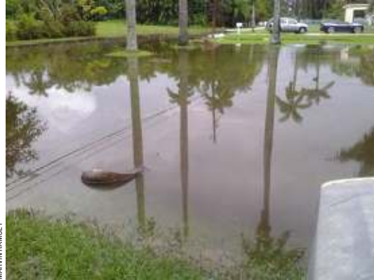
A resident's photos depict floods that are damaging area public spaces, infrastructure, and property.
