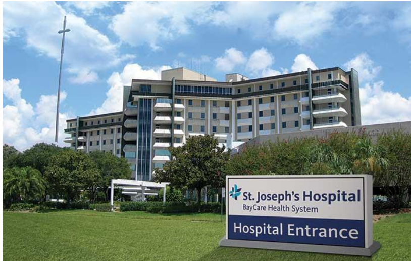
St. Josephs Hospital, Tampa
