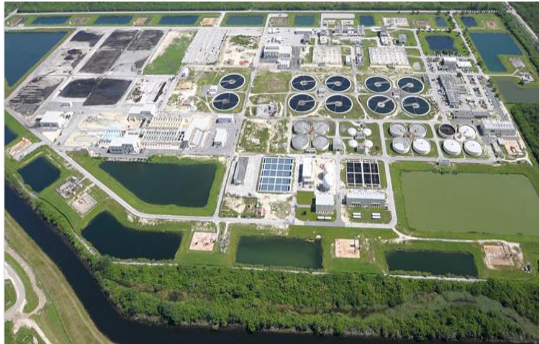
Aerial View of South District WWTP
