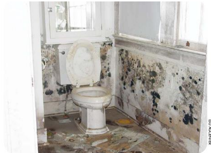
This New Orleans home was flooded for weeks, then sat wet for months before the homeowner was allowed to return and face the results.
