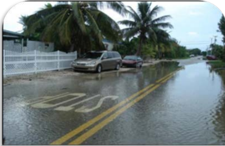
High-tide flooded road on Big Pine Key
