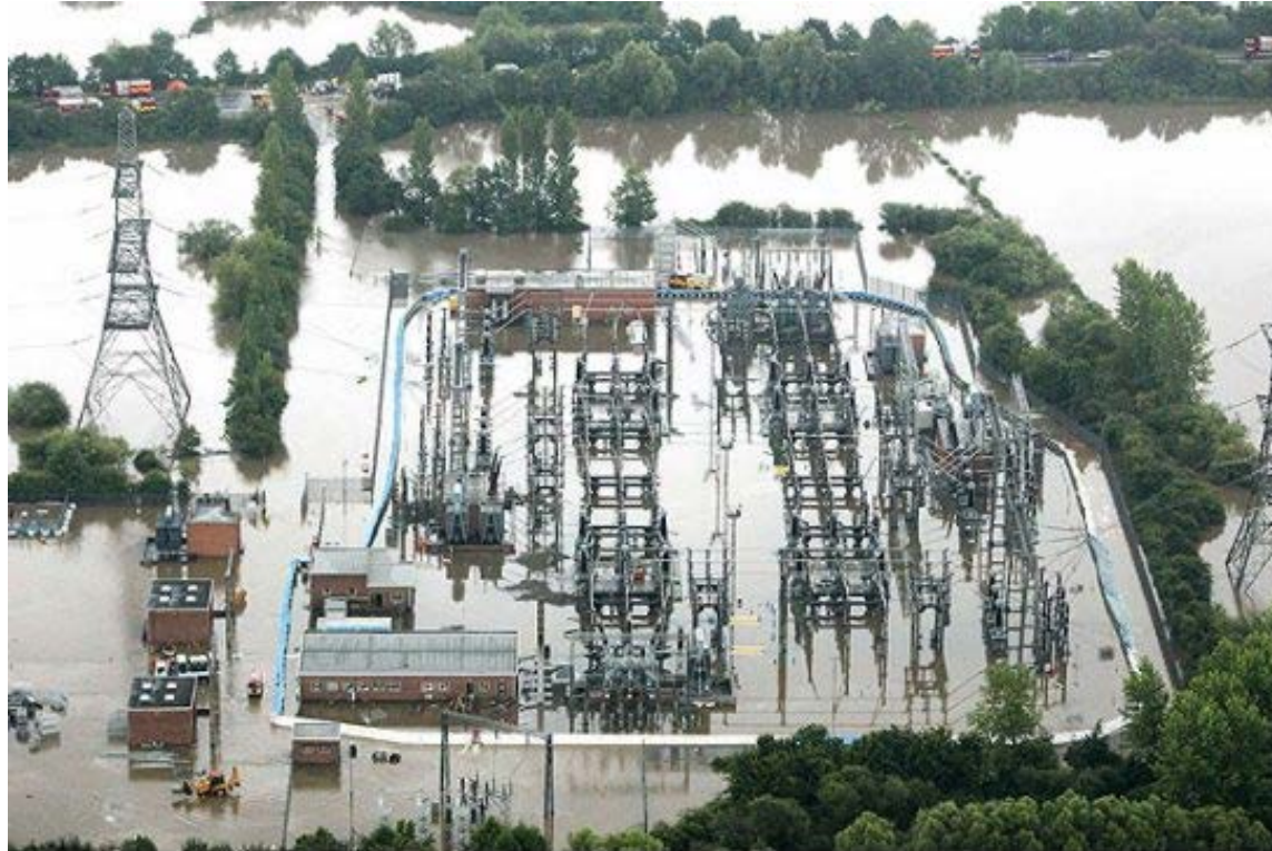
Flooded electrical substation Tewkesbury, England
