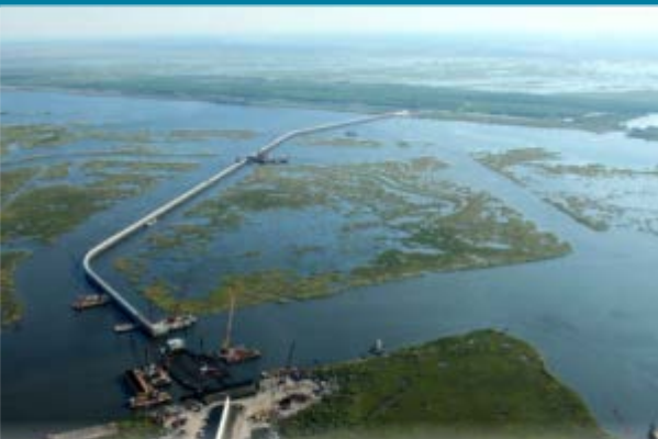
Lake Borgne Storm Surge Barrier
