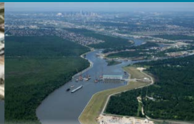
West Closure – Pump Station
